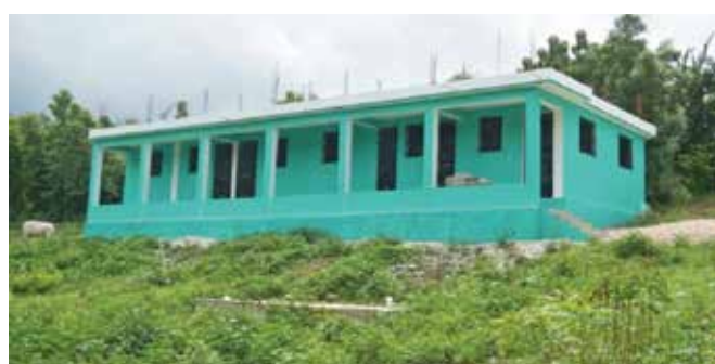
Newly Constructed School Building
