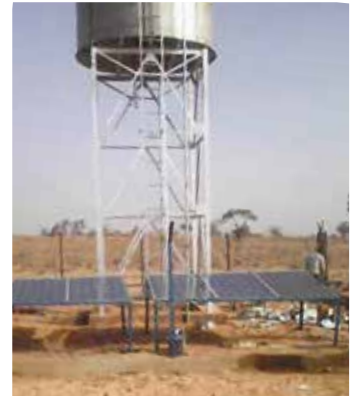
Water Tower with Solar Panels
