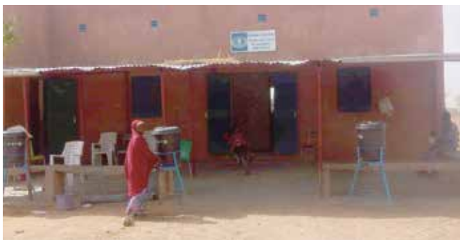
Roof Repair Completed
